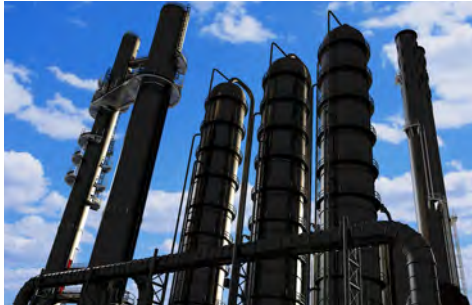
Oil+gas processing and petrochemical complex, Azerbaijan.
