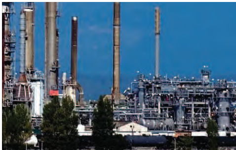
Remediation of a sludge waste lagoon, Italy
